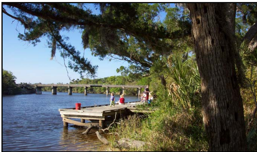
Drawbridge at Highbridge Road
